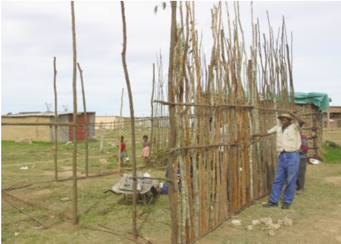
Building a house.
