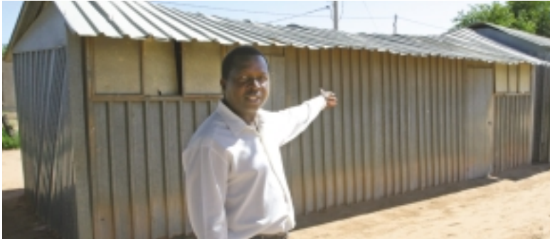
The classrooms built of corrugated steel.
